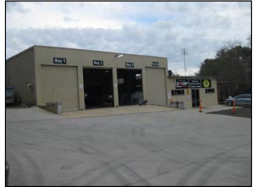
Photograph 6: The workshop, office and hardstand area.
