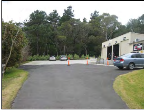
Photograph 5: The workshop building to the east of the dwelling.
