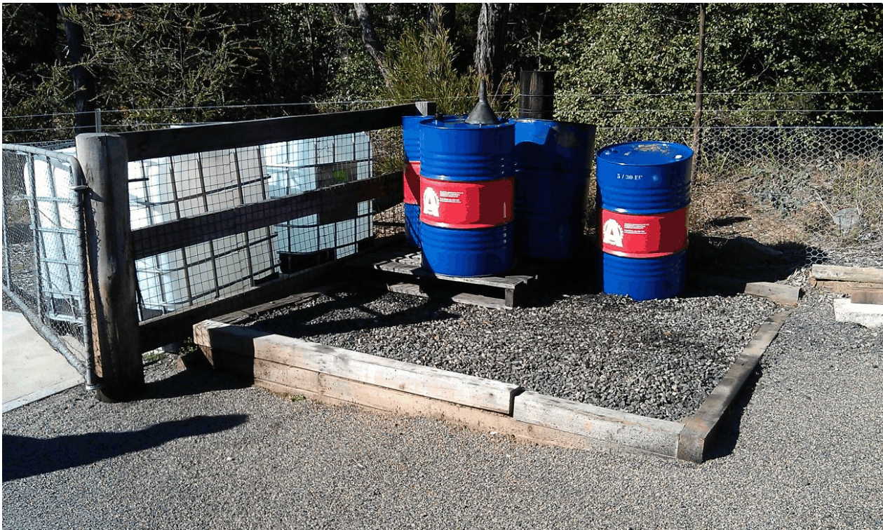
Figure 5 - Used-oil containers on an unsealed, un-bunded surface (both steel and plastic)
